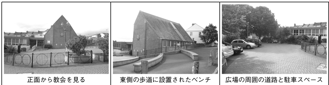
Figure 4. Photos of Balfour Terrace
